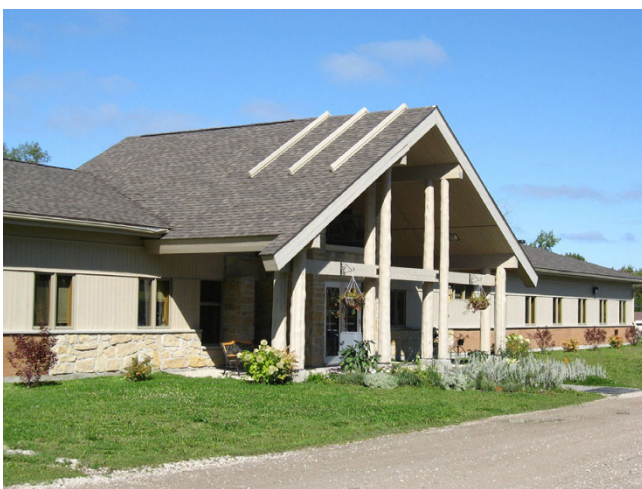
Figure 1 The Share Office Building.
